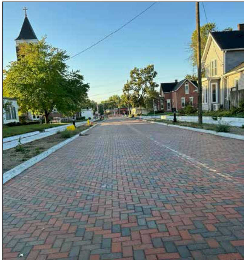
The historic Yandes Street was restored. (Submitted photo)
