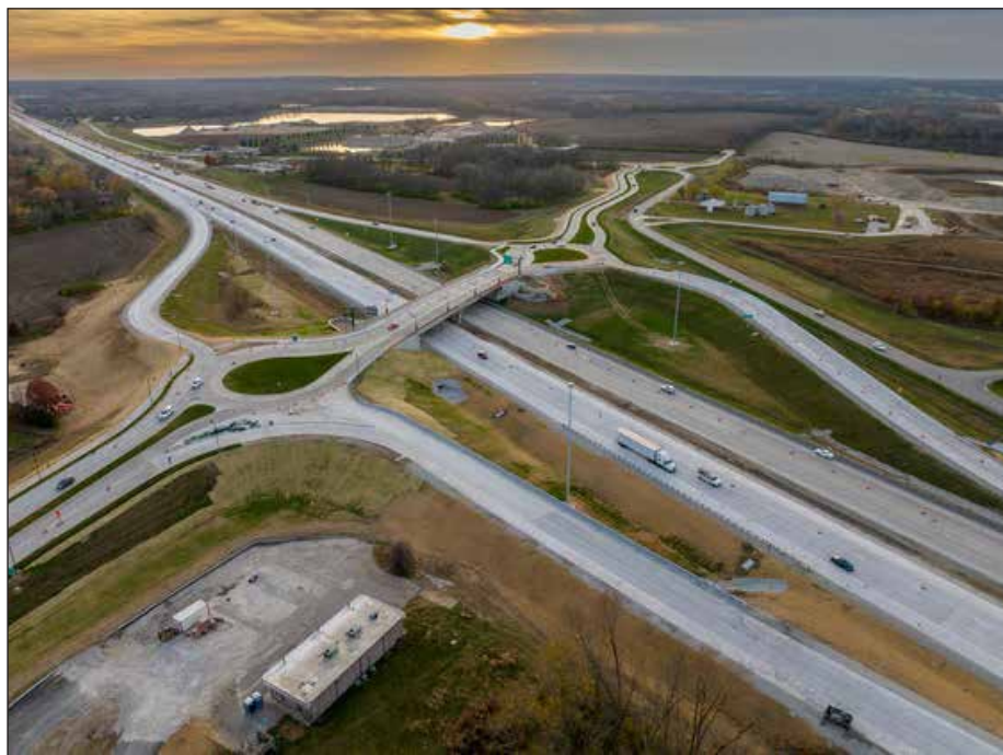
I-69 Construction. (Photo courtesy of INDOT)
