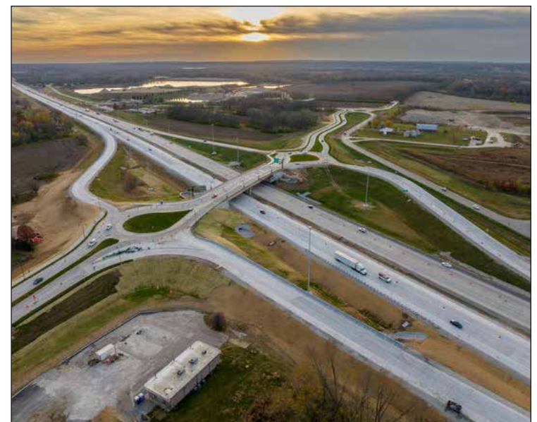
I-69 Construction. (Photo courtesy of INDOT)
