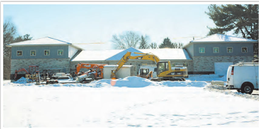
The Southport Municipal Complex is under construction. (Photo by Nicole Davis)
