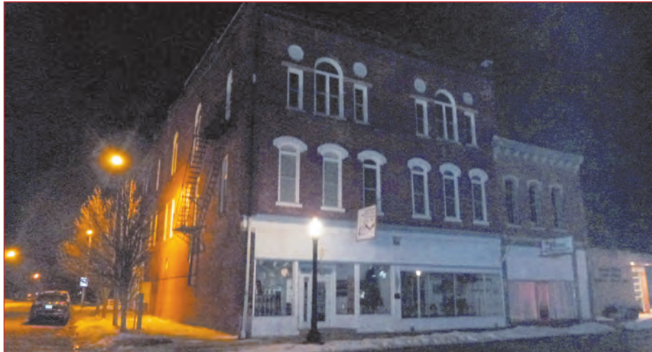
The second floor and an appointment with a shadow figure. (Photo by Rick Hinton)
