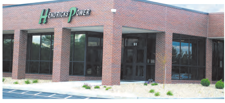
Hendricks County Power Cooperative, 86 N County Rd 500 E, Avon.
