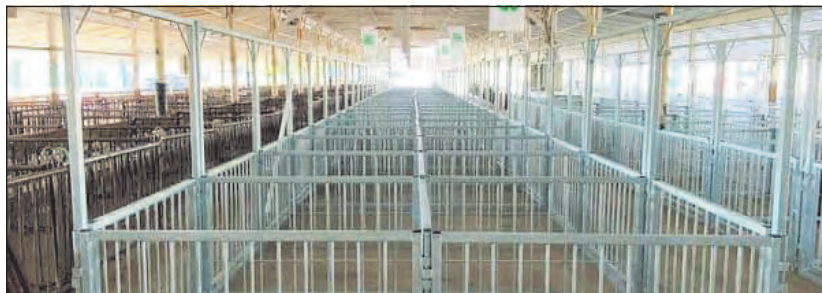
Johnson County Fairgrounds is renovating 300 total swine pens. (Submitted photo)
