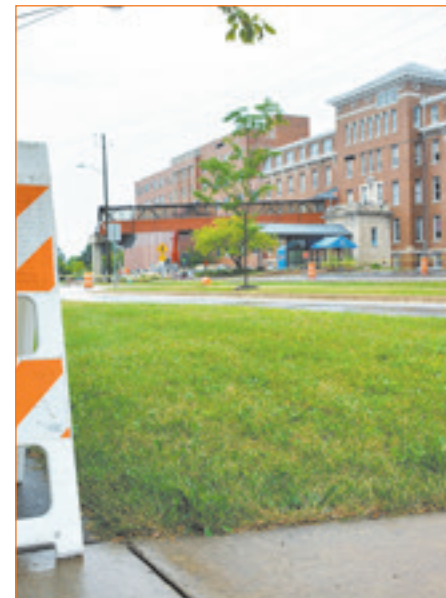
Construction that took place at the old St. Francis in 2015.
