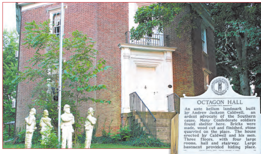
The front entrance of Octagon Hall. Behind the front steps is an alcove once used to hide Confederate soldiers from visiting Union troops. Inset, welcome to Octagon Hall. Photos by Rick Hinton
