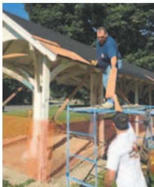
Local 301 volunteers to install wood shakes on a historic trolley house located in Garfield Park.
