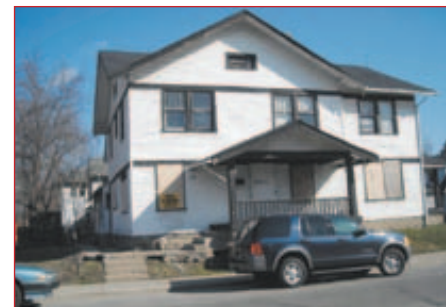
The scene of the crime—3850 East New York Street—shortly before it was bulldozed to the ground.
