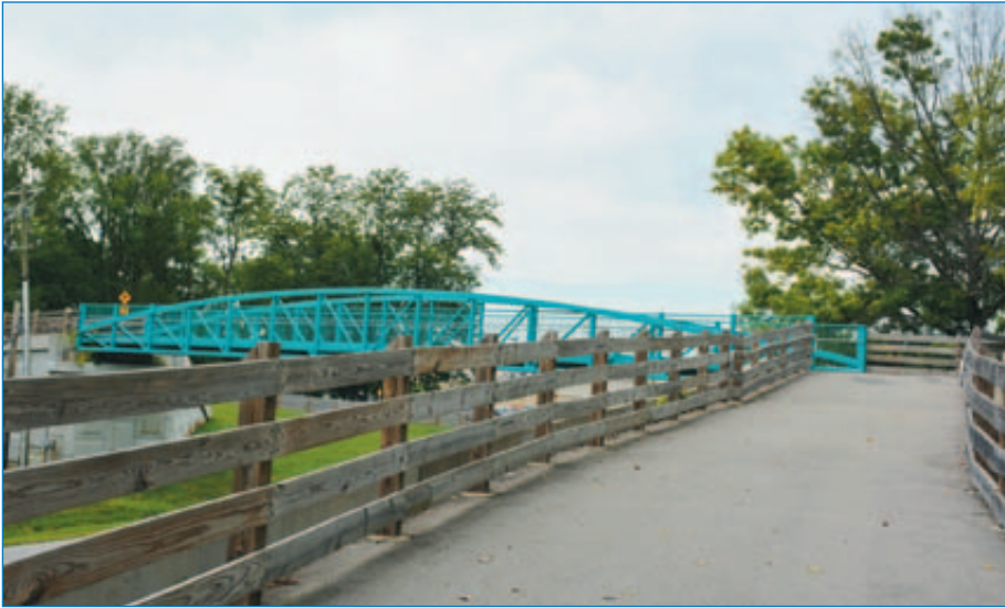
Bridge over Smith Valley Road in Greenwood is part of the Greenwood trail system. Photo by Nicole Davis
