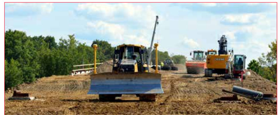
Contractor Superior Construction working the Avon Avenue Bridge Project, Friday, Aug. 25, 2017.
