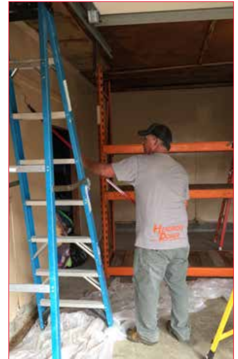
Submitted photo Hendricks County Power Cooperative volunteer helping with renovation.
