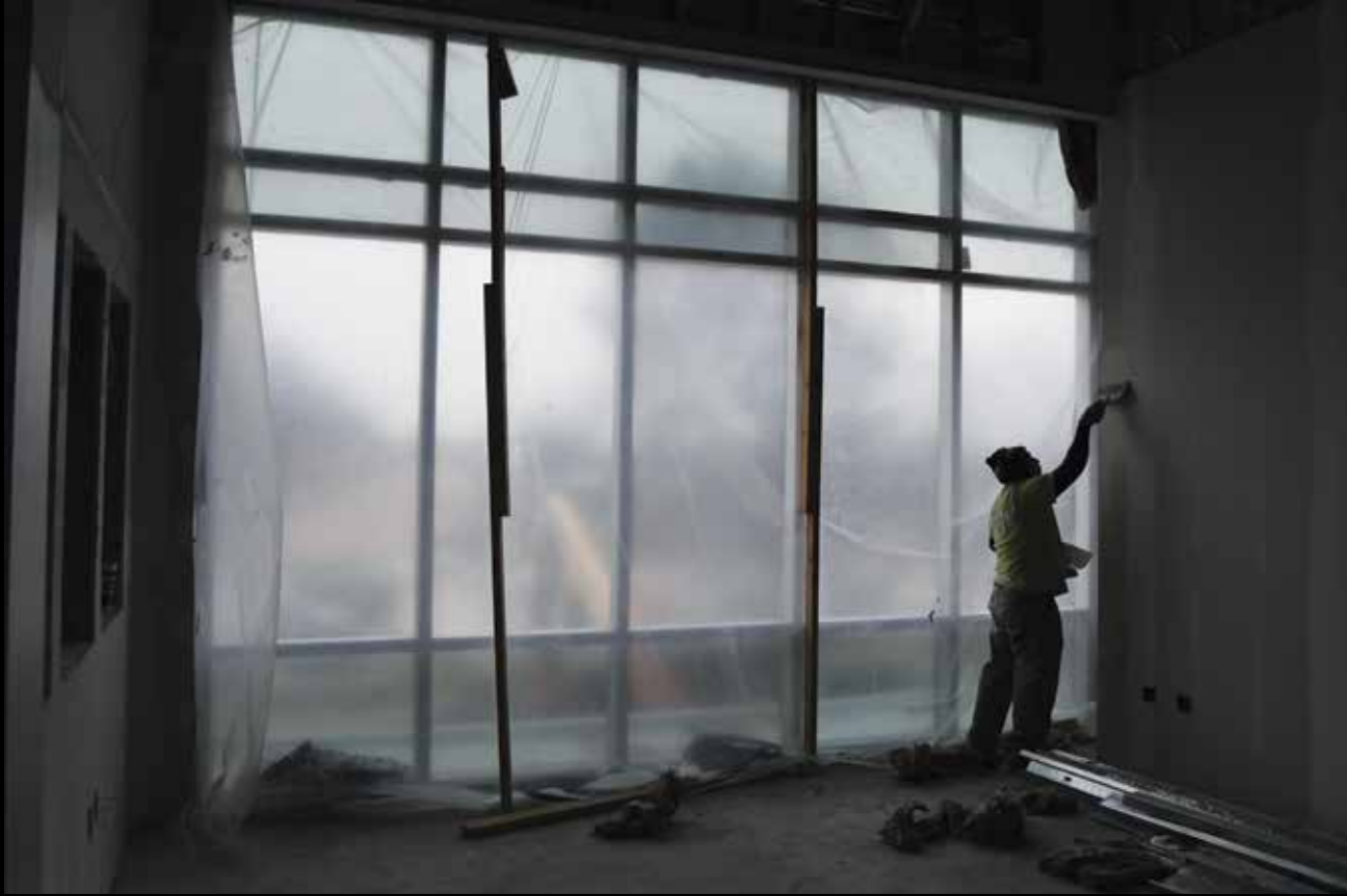
A worker is silhouetted doing some drywall work.
