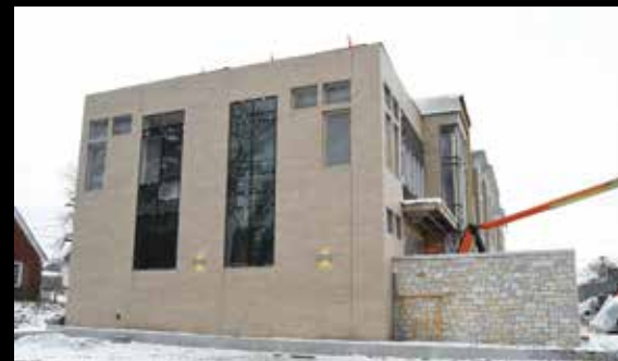
An outside view of the renovations facing west.
